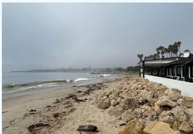
Figure 17: Recently rebuilt Goleta Beach restaurant and cobble berms. Source: Resilient Cities Catalyst. Goleta Beach Site Visit, December 2024
