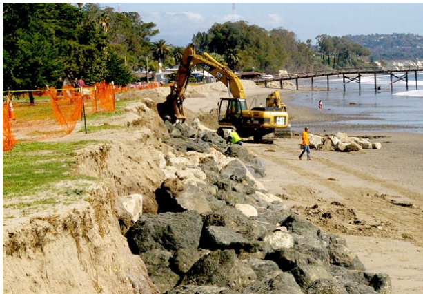
Figure 19: Rock revetment repair through emergency permits to stem storm-caused erosion. Photo Source: Tom Bolton, Noozhawk , 2016.
