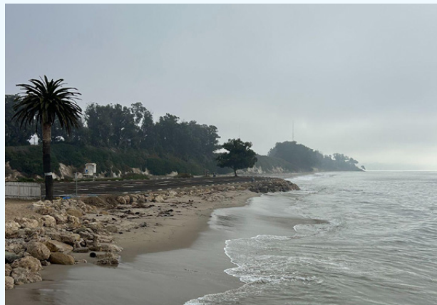
Figure 18: Tides reaching cobble berm around recently rebuilt parking lot. Source: Resilient Cities Catalyst. Goleta Beach Site Visit, December 2024
